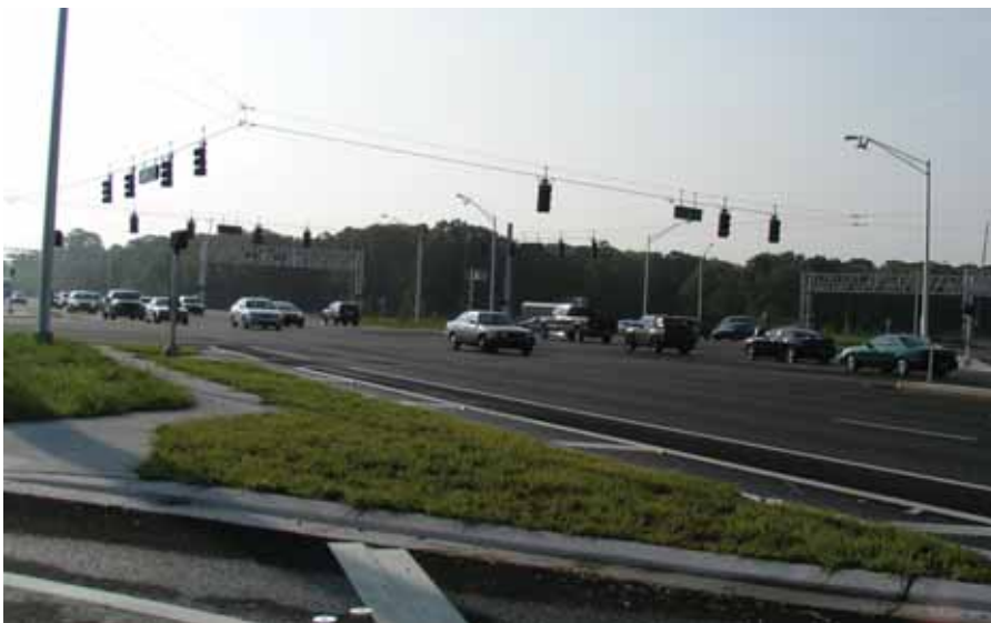
Looking southeast highlighted by the "suspended box" signal configuration, which includes video vehicle detection, railroad and emergency preemption, illuminated street name signs, and signalized pedestrian crossings.
