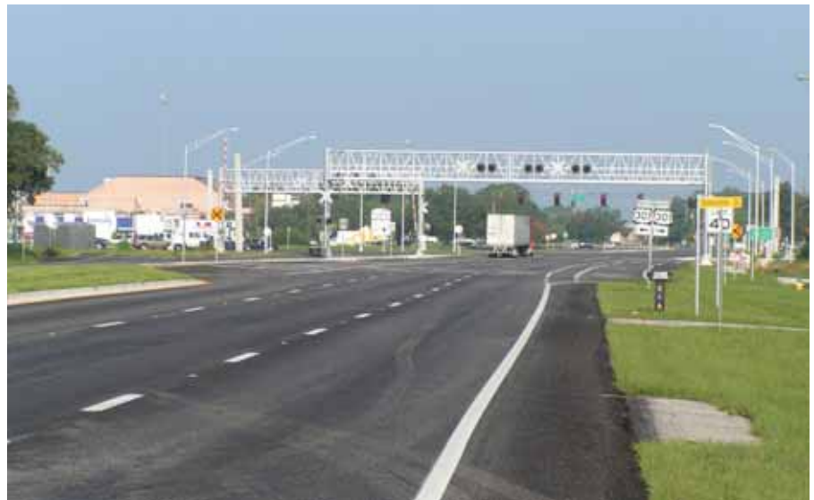
A westbound view of University Parkway in Sarasota, Fla., highlighted by improved railroad crossing bridge structures for two crossings, along with improved turn lane capacity.
