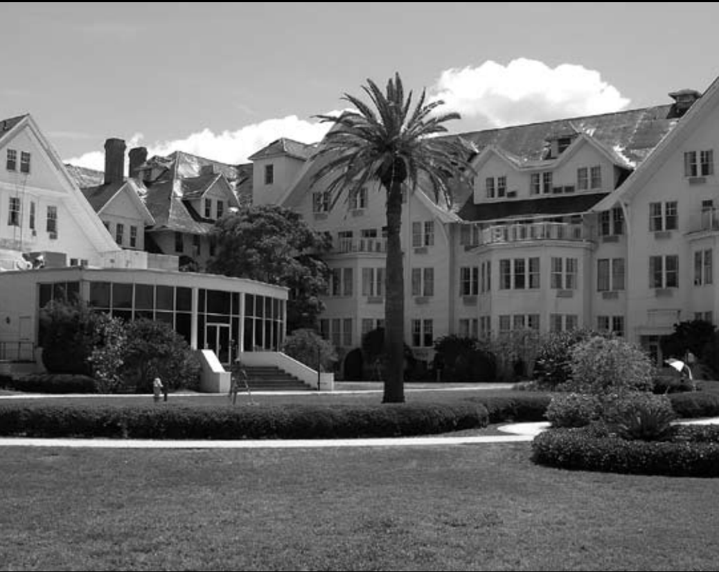
SURVEYORS WERE ABLE TO COLLECT AS-BUILT DATA OF THE ENTIRE HOTEL AND THREE COTTAGES DURING A TWO-WEEK PERIOD WITHOUT CLIMBING THE STEEP ROOFS AND GABLE DORMERS.
