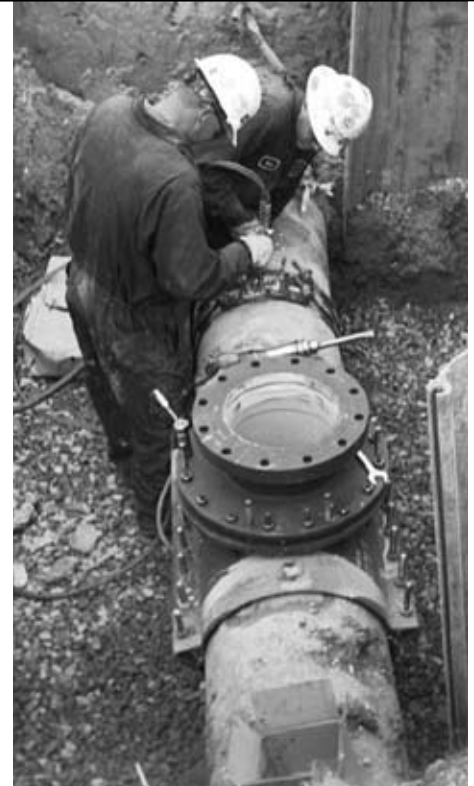
PIPE FITTINGS ARE INSTALLED (ABOVE) ON EITHER SIDE OF A VALVE TO ENABLE THE LINE STOP (BELOW) TO ISOLATE THE AREA FOR REPAIR.
