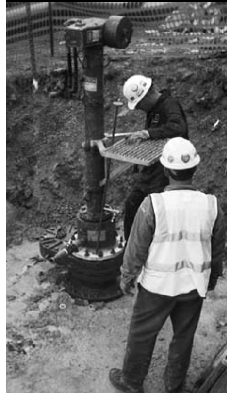
PIPE FITTINGS ARE INSTALLED (ABOVE) ON EITHER SIDE OF A VALVE TO ENABLE THE LINE STOP (BELOW) TO ISOLATE THE AREA FOR REPAIR.
