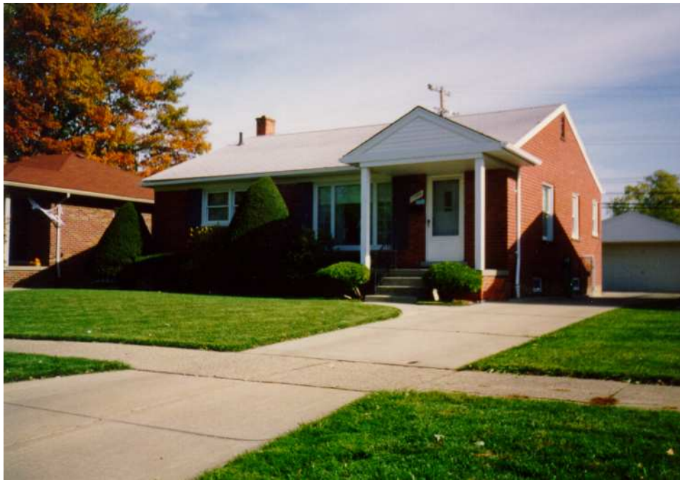
Standard one-story brick ranch in good structural condition.
