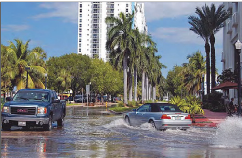
“Sunny day” flooding in Sunset Harbour prior to improvements.
