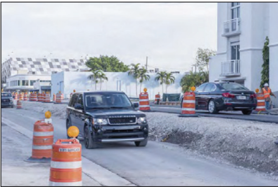
Sunset Harbour roadway during elevated roadway construction.
