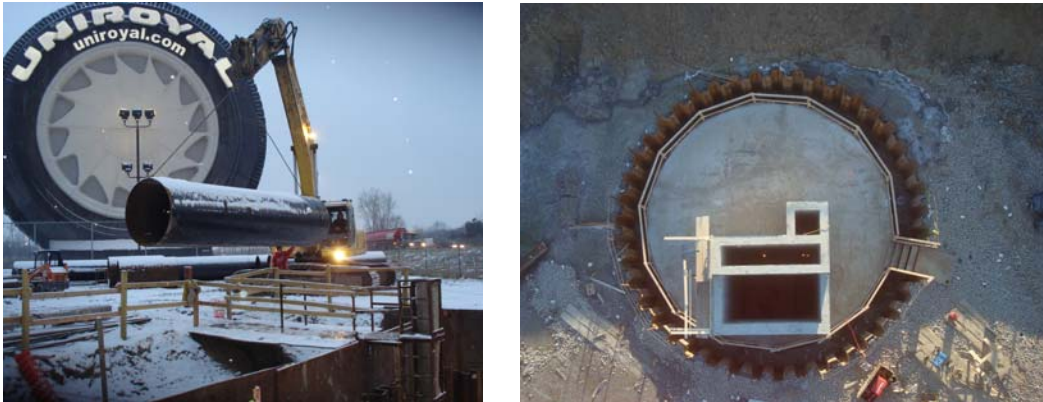
Figure 4. Each shaft location presents unique challenges
