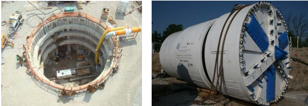
Figure 5. Secant pile shaft and TBM prior to insertion
