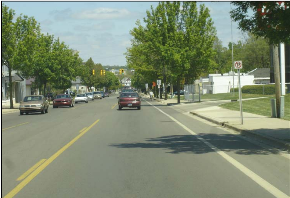
After – Capital Avenue Two Lanes with Center Turn
