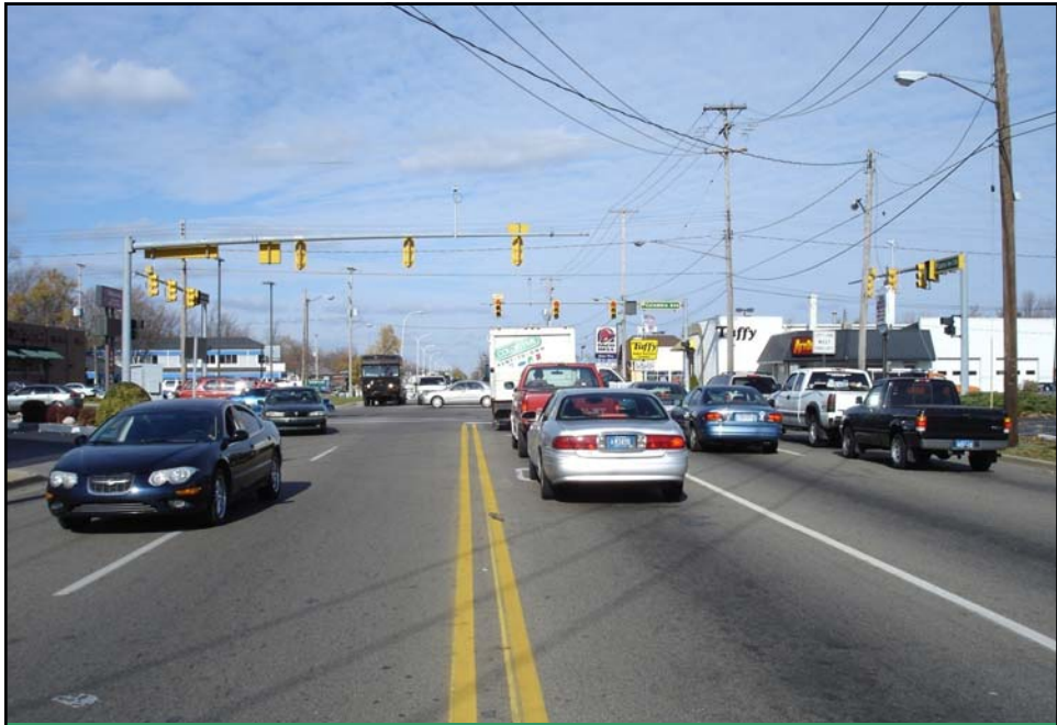
Before – Capital Avenue at Columbia
