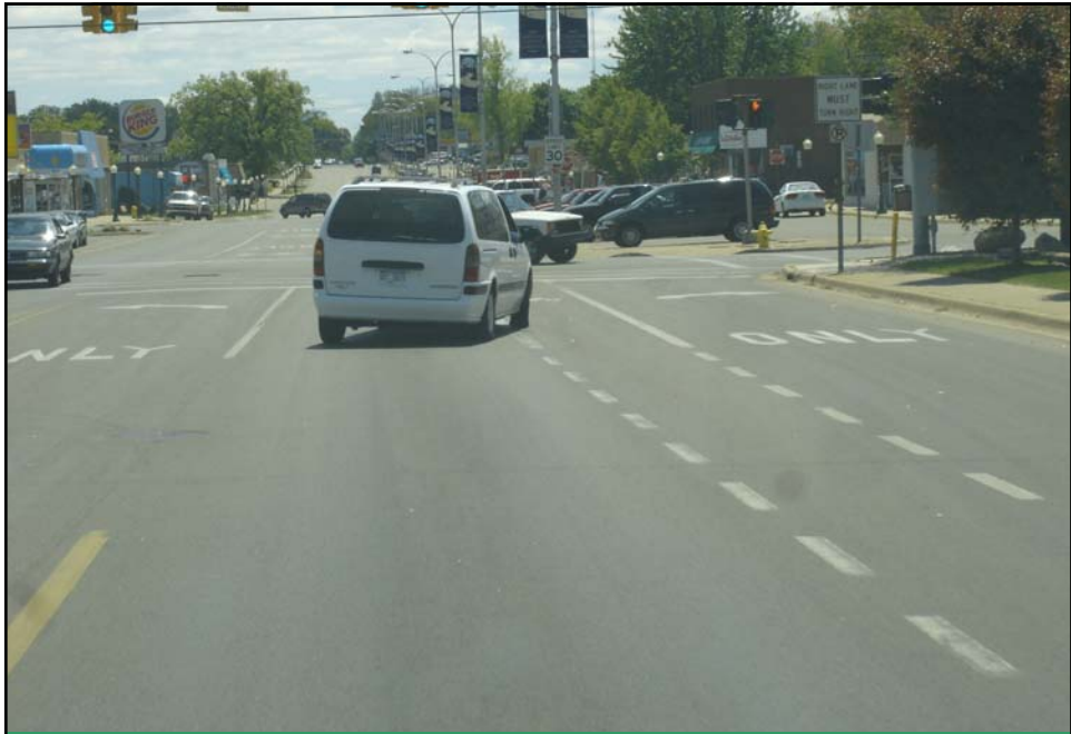
After – Capital Avenue SW at Territorial Road
