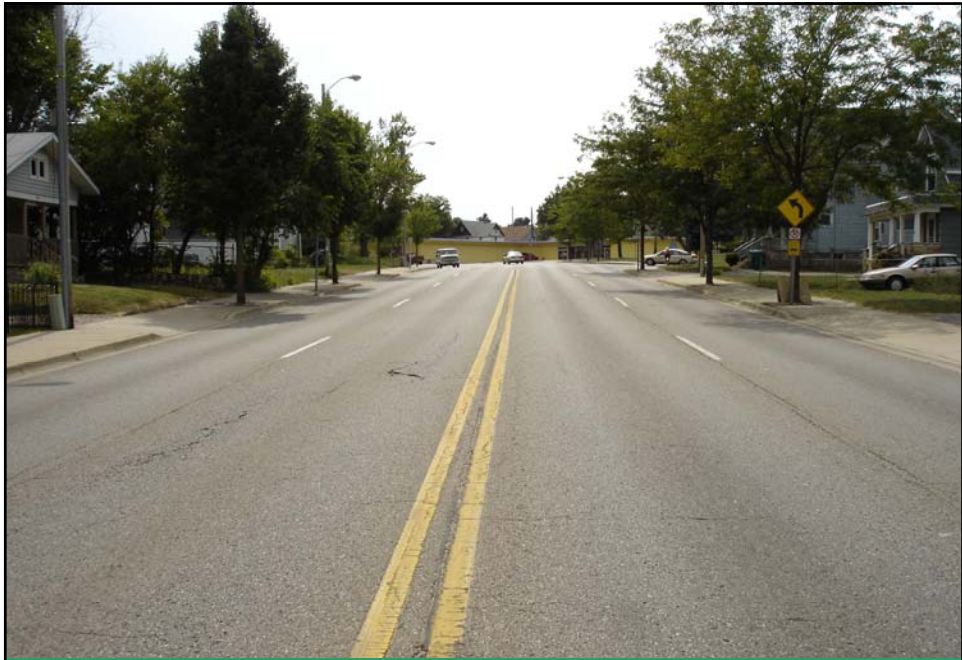
Before – Capital Avenue Four Through Lanes
