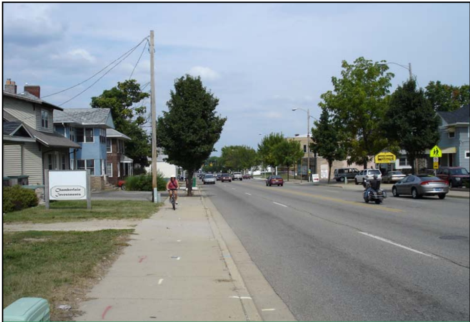
Before – Capital Avenue Four Through Lanes
