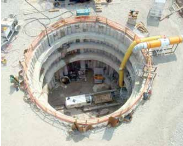
Secant pile shaft and TBM prior to insertion.
