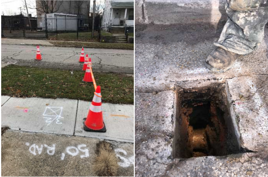
Figure 6: Example SUE Quality Level A Investigation
