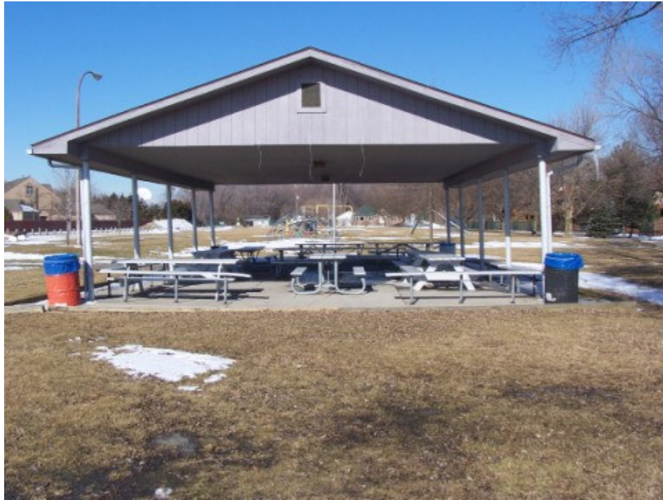
Photograph No. 14: Looking west at shelter.
