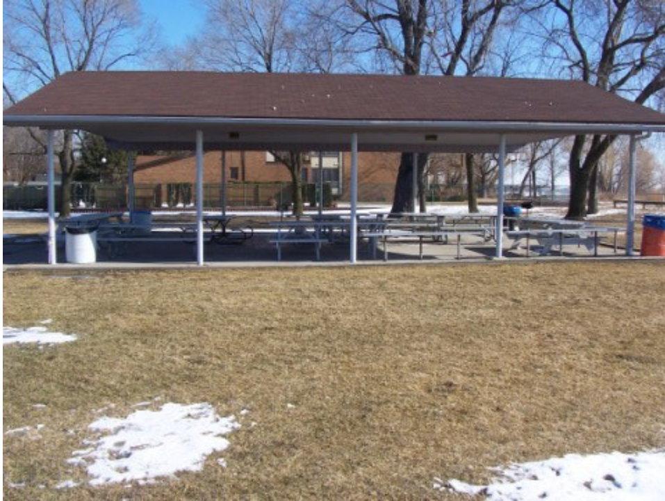
Photograph No. 1: Looking north at shelter.
