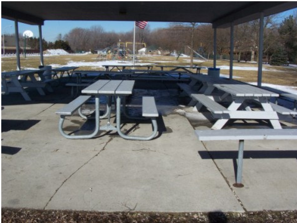
Photograph No. 16: Looking west at shelter.
