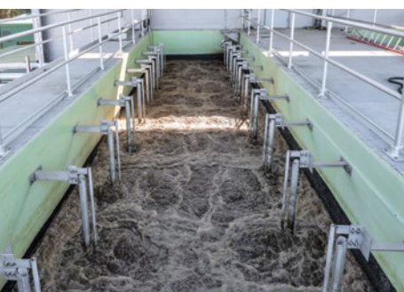
The revived Travis Field facility uses membrane bioreactor technology to treat wastewater to reclaimed standards.
