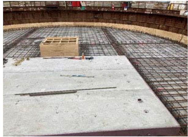
Figure 18. DVT-2 top slab structure layout
