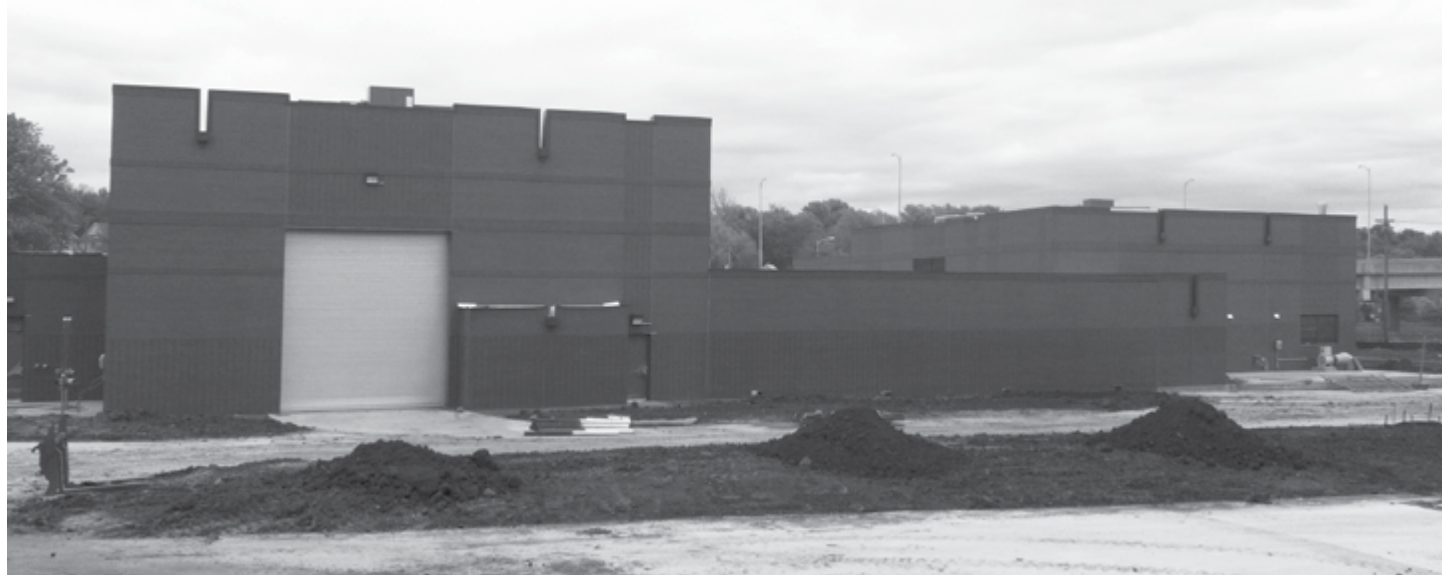
The SOIA Lift Station includes a Screen Building (left), Odor Control Enclosure (middle), and a Pump Building (right).
