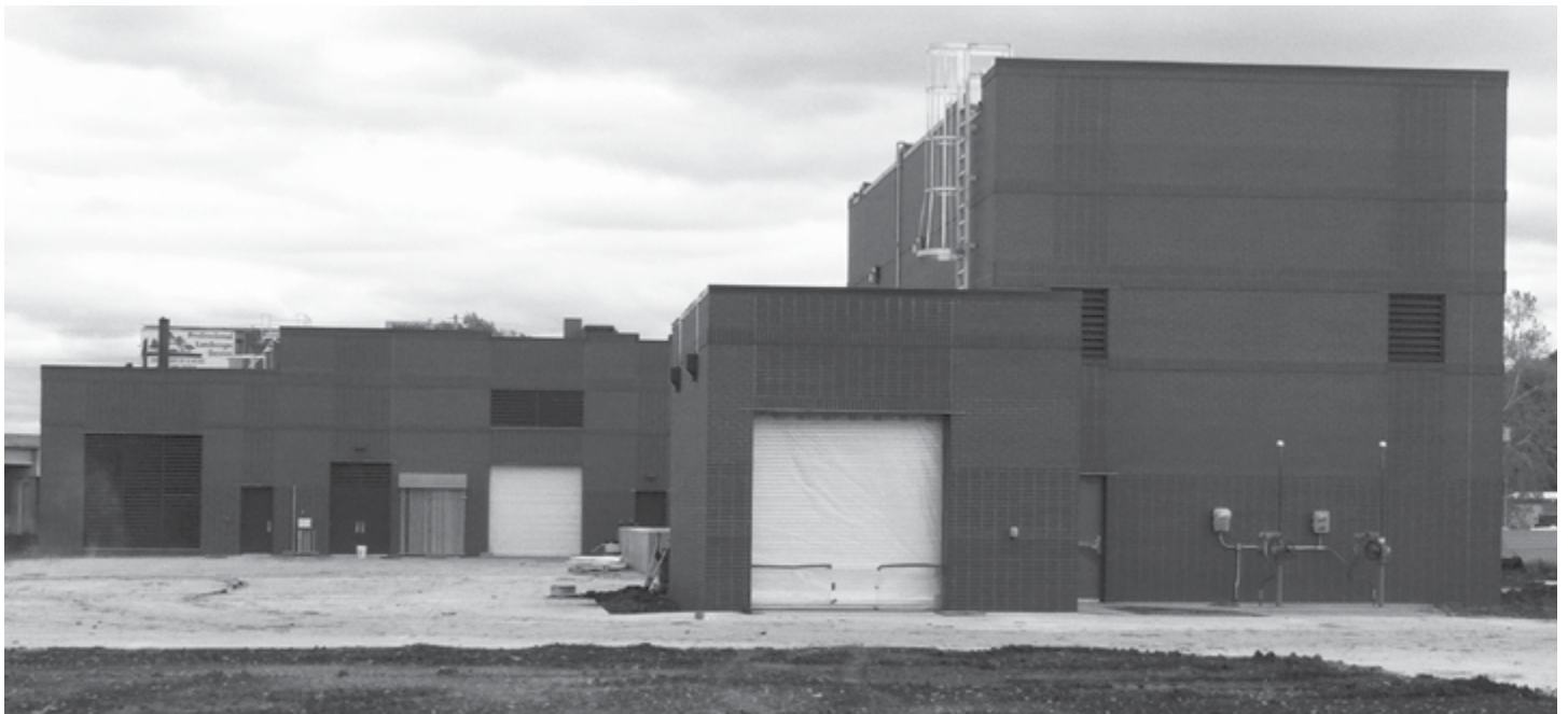
A courtyard behind the lift station provides access to the main working areas and screens most maintenance activities from the view of nearby residents and businesses.
