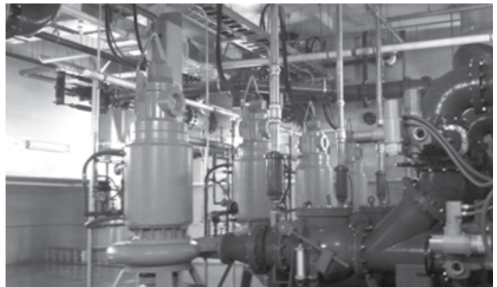
Each of the four dry pit submersible pumps will deliver up to 4,000 gpm.
