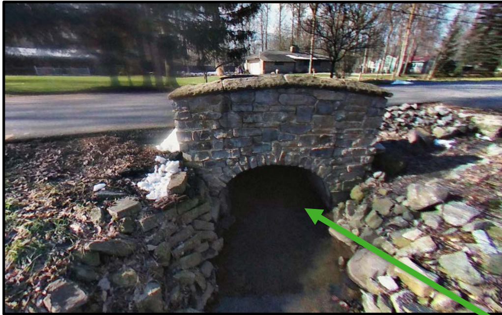
Spherical Imagery of culvert
