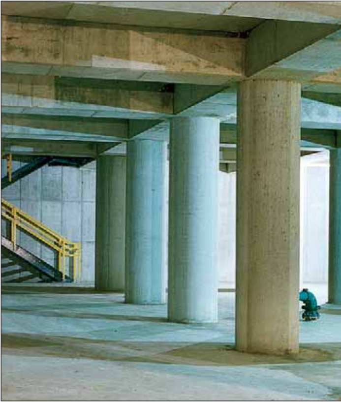
New design criteria, based on expected future performance of SSO control rather than a hypothetical 25-year design storm, was developed with MDEQ to determine the equalization basin's storage volume, resulting in a cost-effective solution that meets regulatory objectives.
