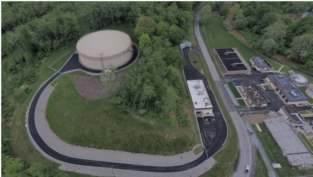
Figure 8: Aerial view of the completed project.
